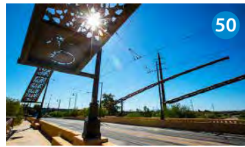
Luis G. Gutierrez Bridge, 2012 Cushing Street Artist: Brenda Semanick and Structural Grace Inc. Architect: Dave Dabler
